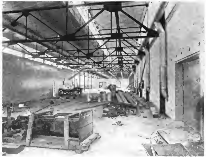
Ready for the final touches, Perlman rim plant in Jackson, Mich.
